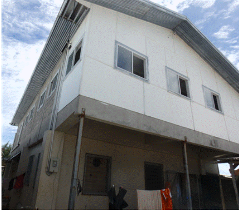
Figure B-7: Jail building in poor condition
