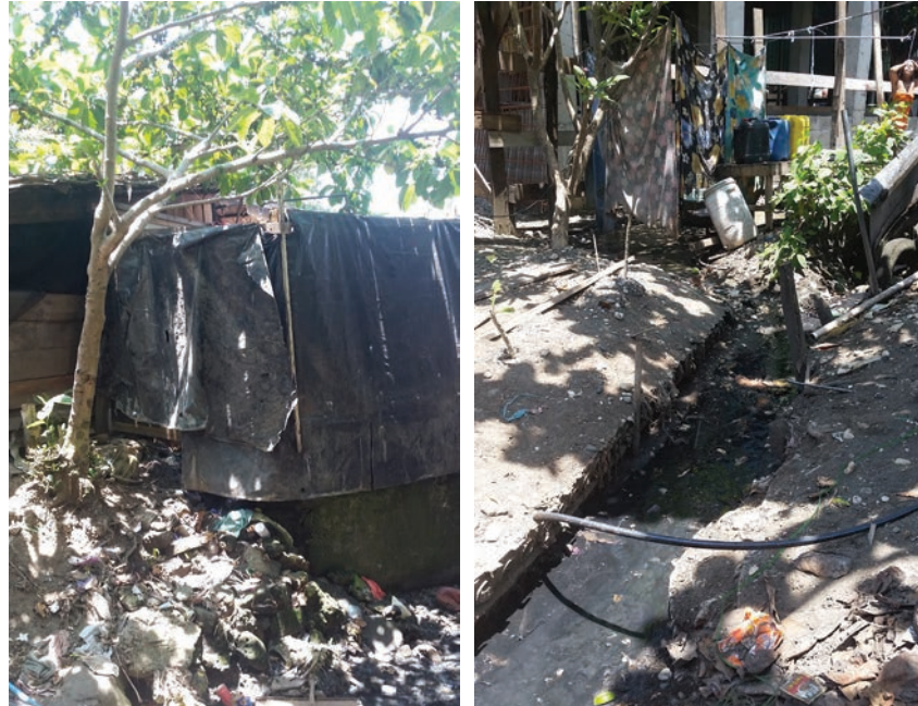
FIGURE 2.1: POOR SOLID WASTE MANAGEMENT AND DRAINAGE IN LORD HOWE SETTLEMENT, HONIARA
