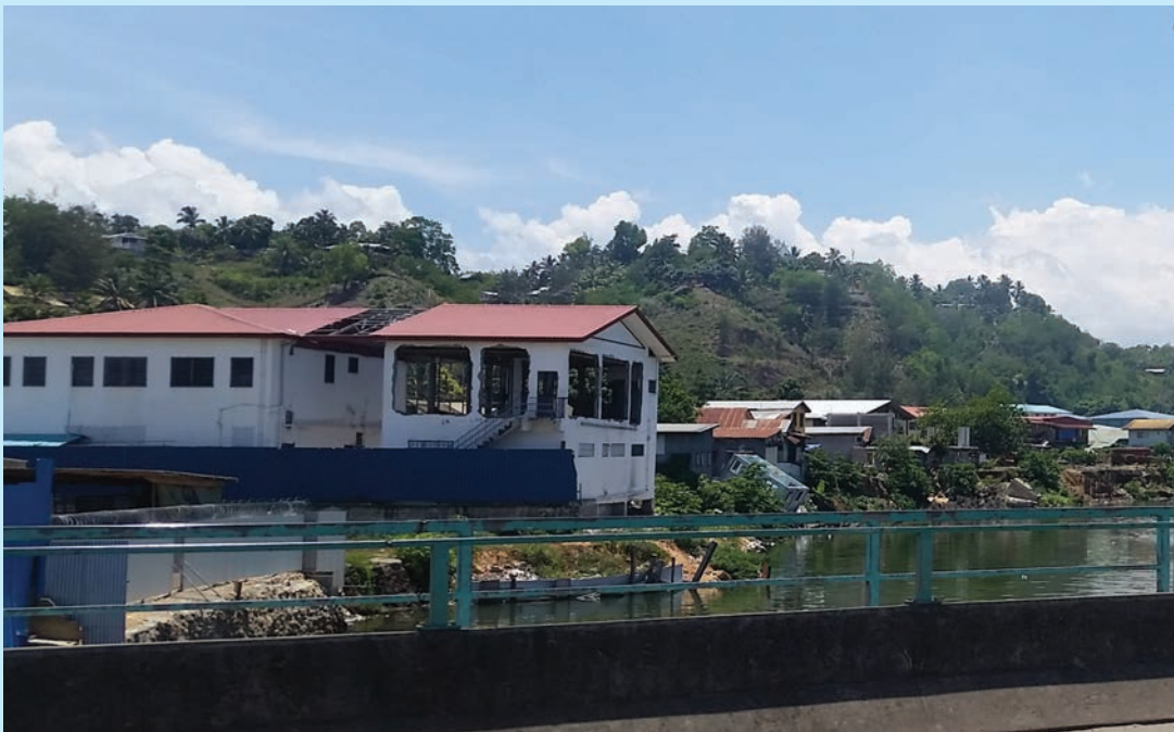
FIGURE 4.2: RE-BUILDING HOMES ALONG THE MATANIKA RIVER IN HONIARA AFTER THE FLOODS
