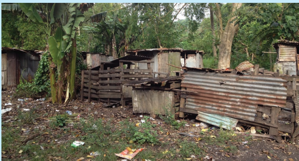
FIGURE 3.11: CURRENT TOILET FACILITIES IN BLACKSANDS SETTLEMENT
