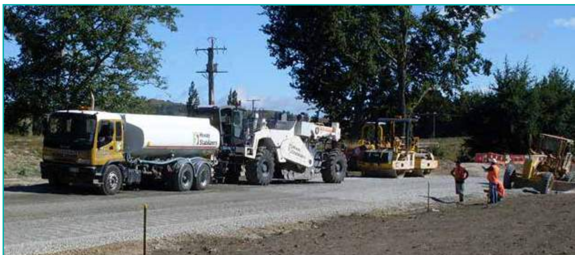
Figure 18. Pavement Stabilising 'Road Train'
