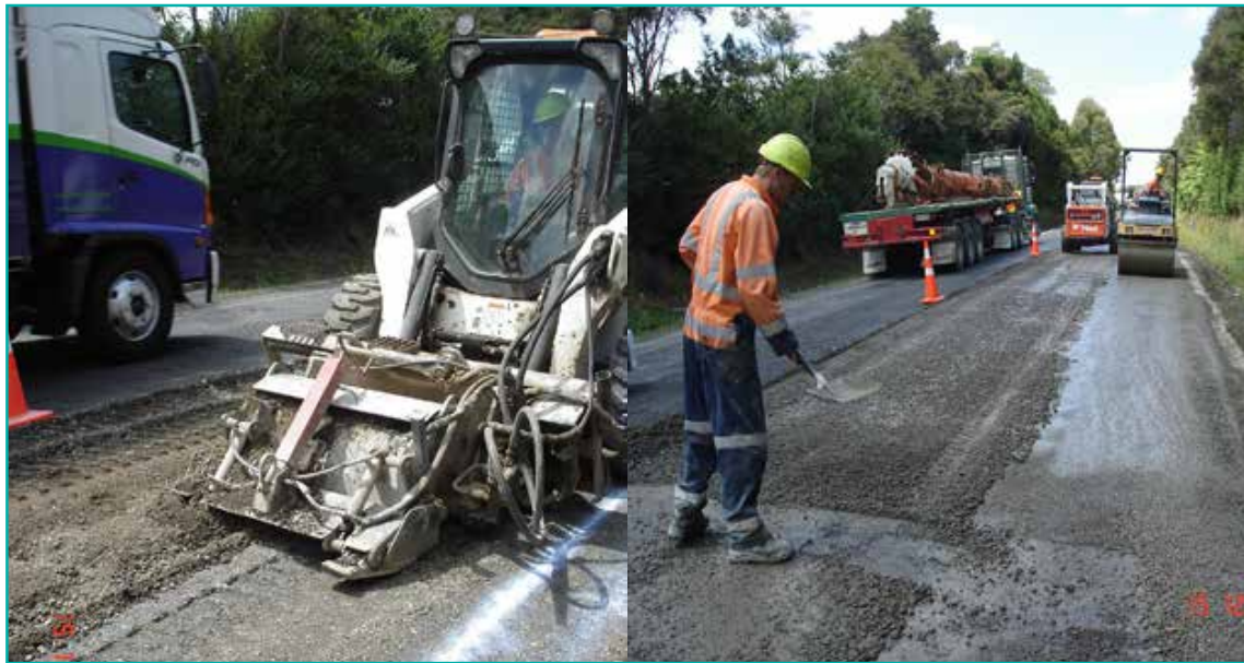
Figure 19. In-situ Aggregate Stabilisation with Small Plant and Skilled Work Crew
