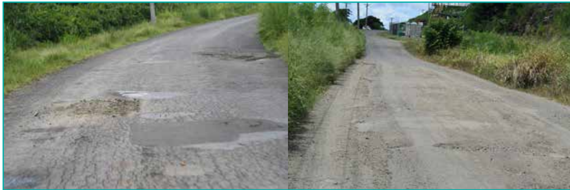
Figure 26. Pavement Project Site in Fiji
