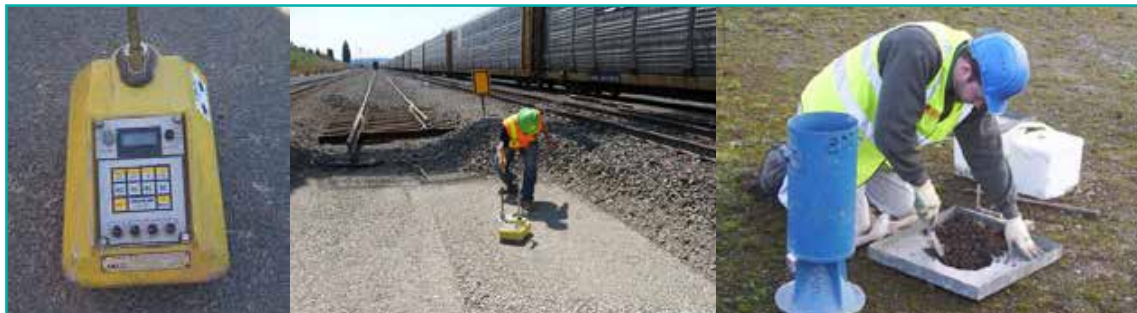
Figure 22. Field Compaction Density Tests
