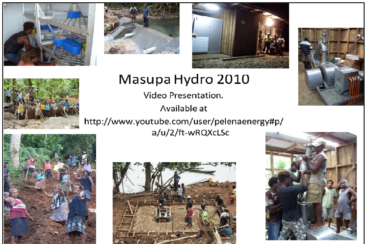
Figure 4: Various photos from the 13-day construction of the Masupa Hydro in Jan/Feb 2010.
