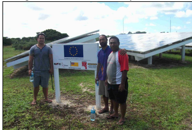
Figure 2.4: Grid-connected PV system in Niue
