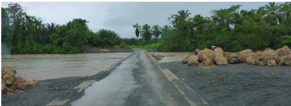
Figure 1: Flooding in Mberande
