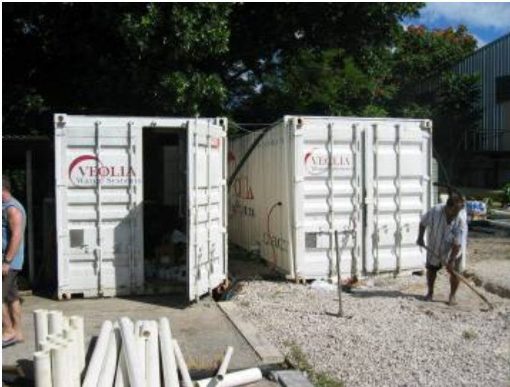
Veolia RO Plant; Model: DS9-C; Output: 120 kL/day per unit.
