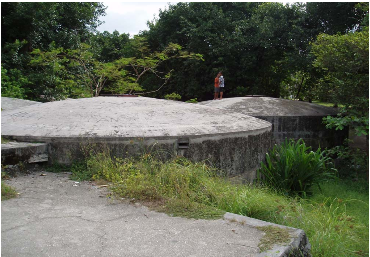
Nauru – Reinforced concrete water storage tanks (derelict)
