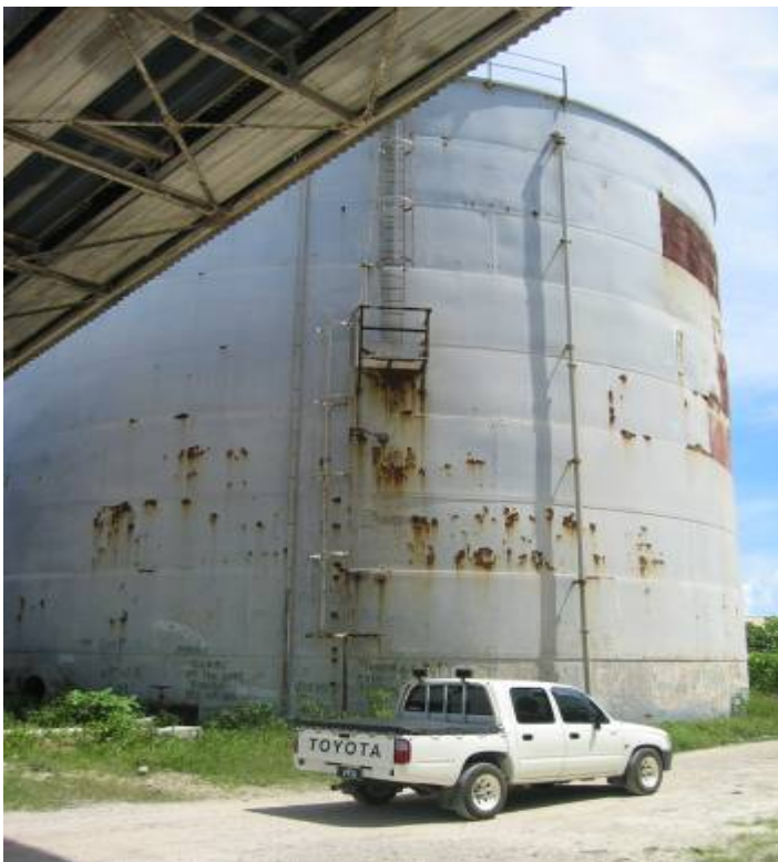
Decommissioned Water Storage Tank B12.
