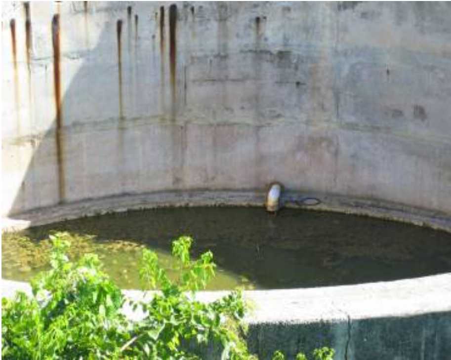
Sea Water Storage Tank Internals
