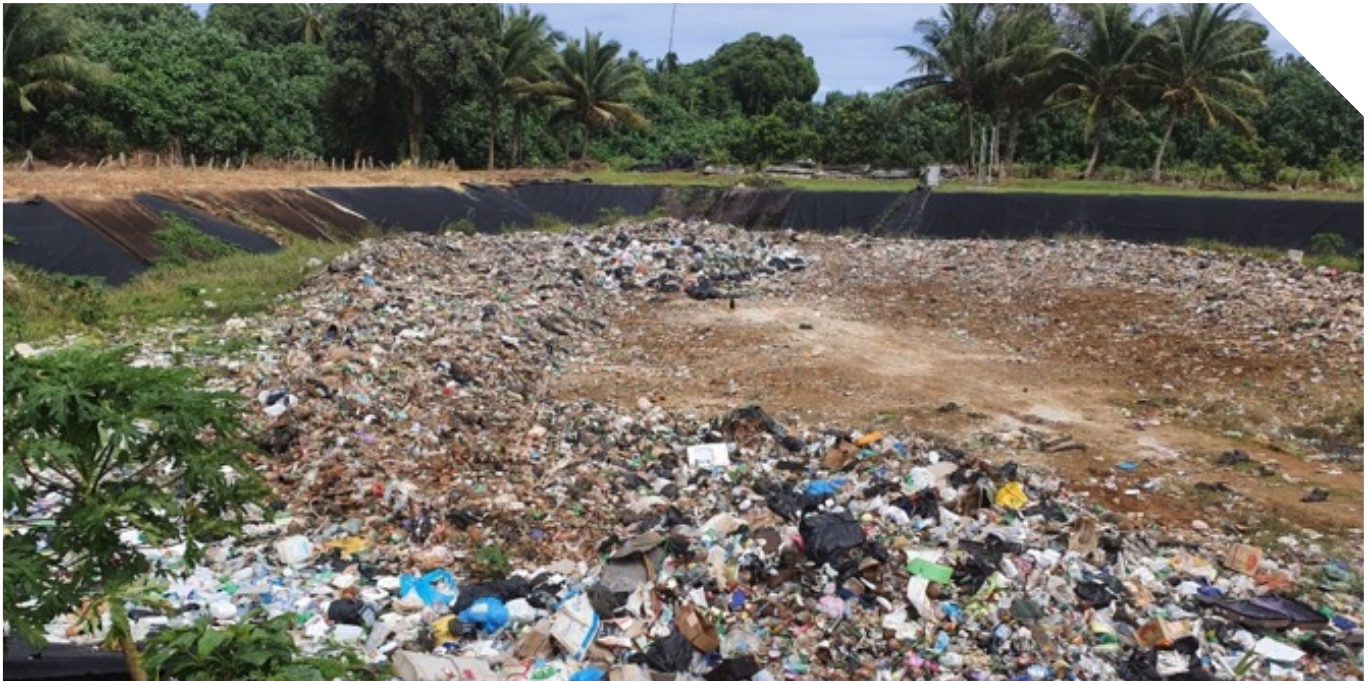
Aitutaki Landfill. The Aitutaki landfill site (photo by Tekao Herrmann, during the waste audit).
