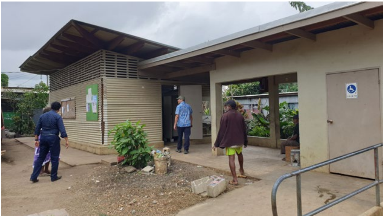
Figure 4-5: Seaside Community Sanitation Project
