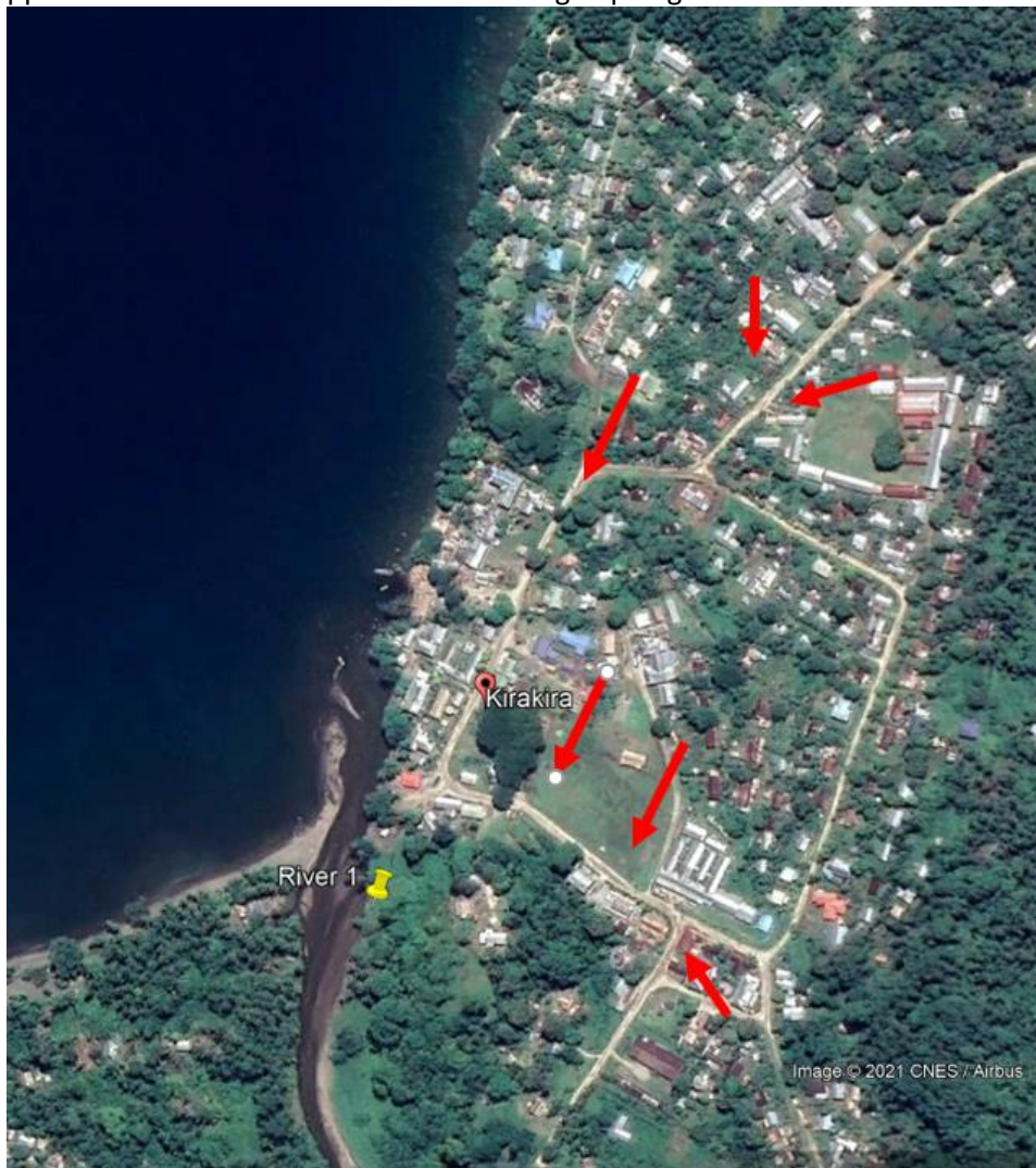
Kirakira Drainage Path
