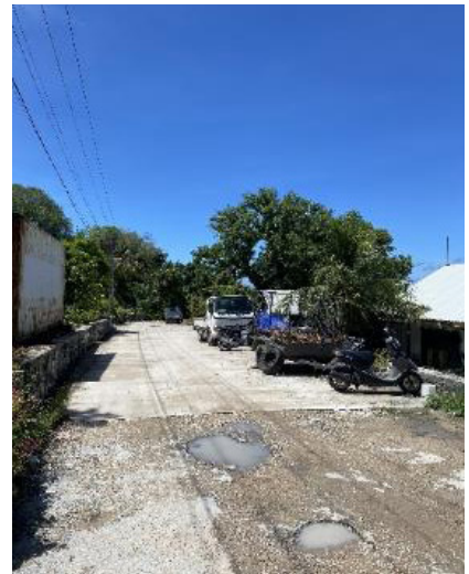
Some road sections have been repaired while adjacent sections have been left as is.
