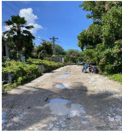
NPC Road condition where no repair work has been done.
