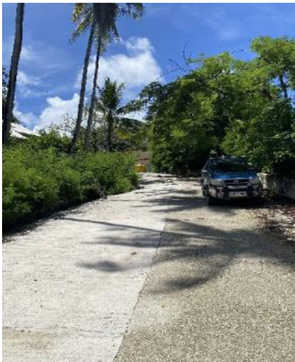
Some road sections have been repaired while adjacent sections have been left as is.
