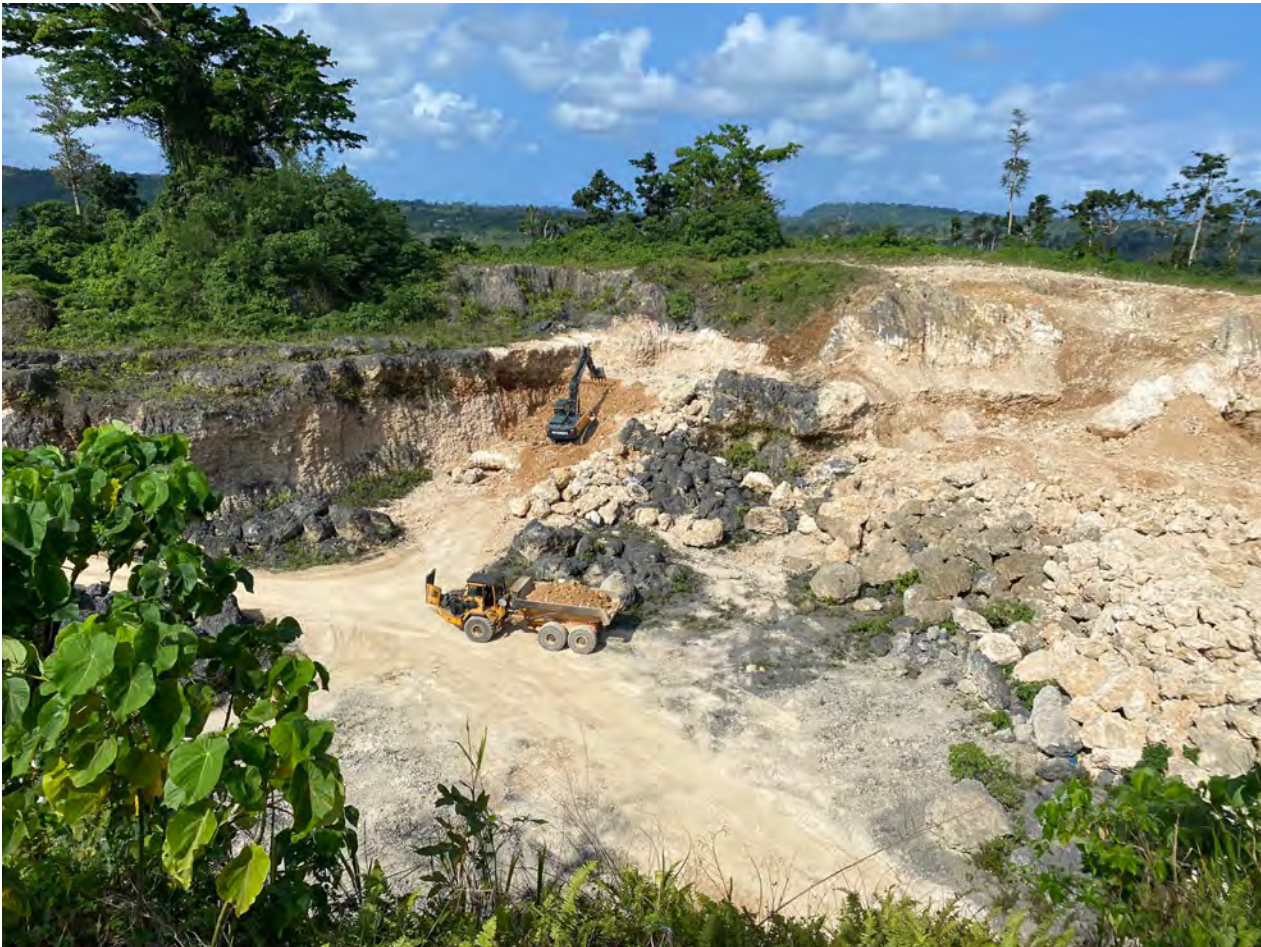
Figure 81: Commercial Limestone Quarry in Efate
