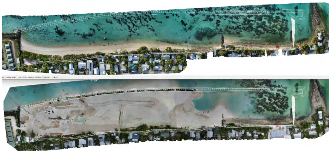
Figure 108: Tuvalu Coastal Adaptation Project (TCAP) on the Capital Fogafale to Protect Communities from Sea-Level Rise
