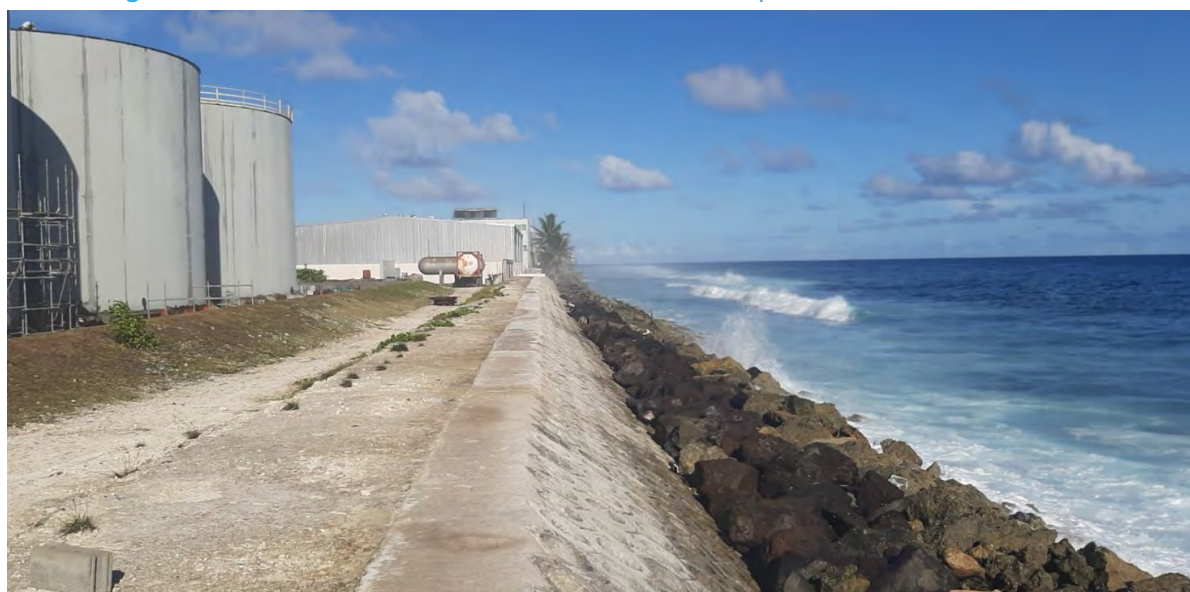
Figure 50: Armor Rock for Coastal Protection in Majuro, the Marshall Islands
