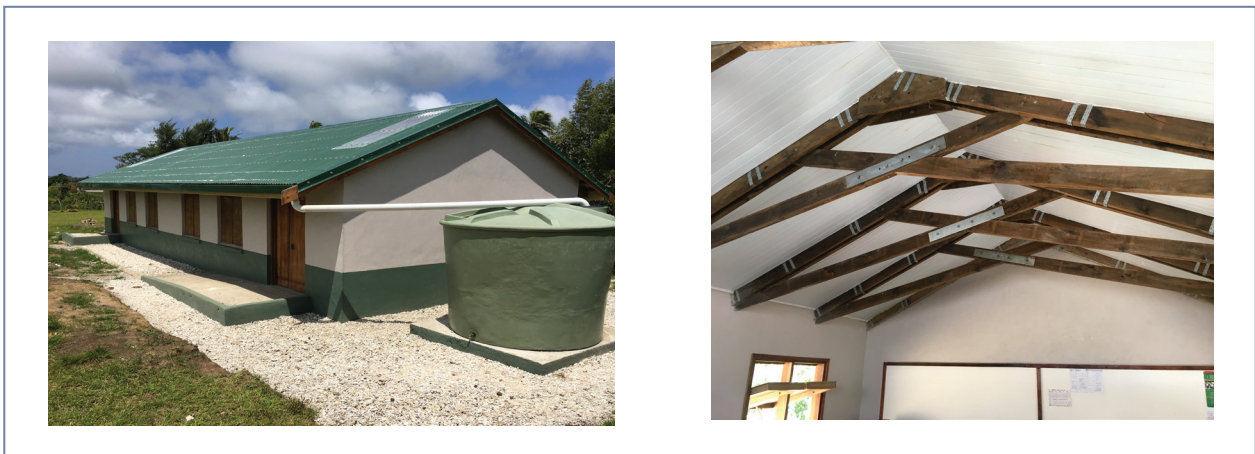
Figure 2-3: Classrooms constructed after Tropical Cyclone Pam in accordance with the National Building Code
