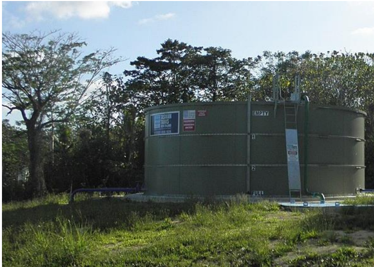
Figure: New Water Tank in Alofi
