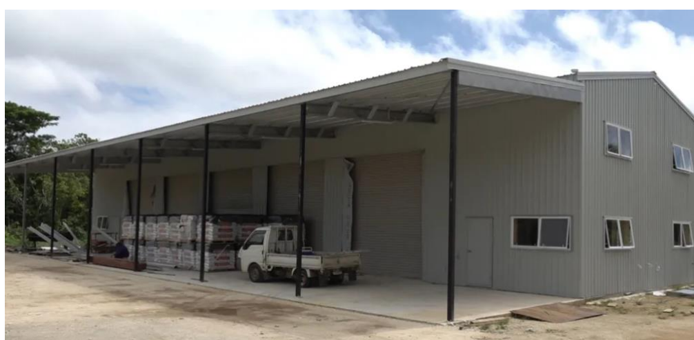
Figure: New Power Station Building
