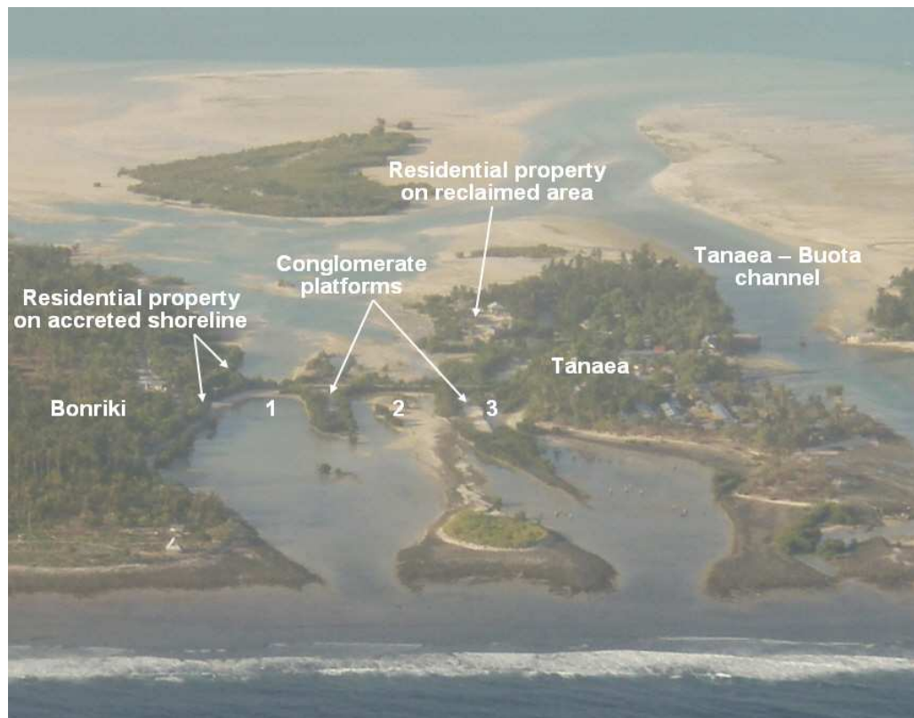
Figure 9: Key features of the Bonriki-Tanaea channel and causeway showing the three sections (numbered 1, 2 and 3) that make up the channel
