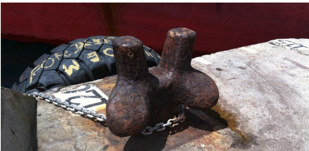
Figure 25 - Bollards at main wharf requiring replacement
