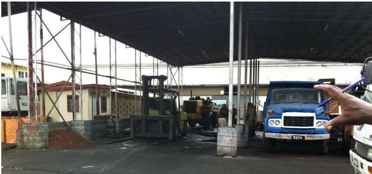
Figure 16 - Plant workshops in secure port operations area
