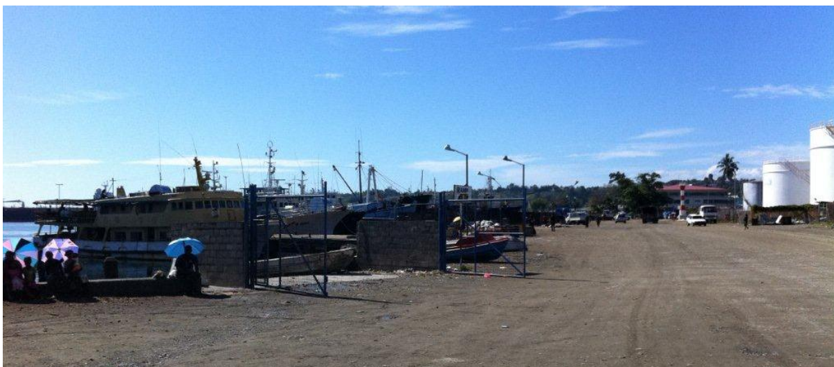
Figure 20 – Access road to coastal jetties and ramps – looking east
