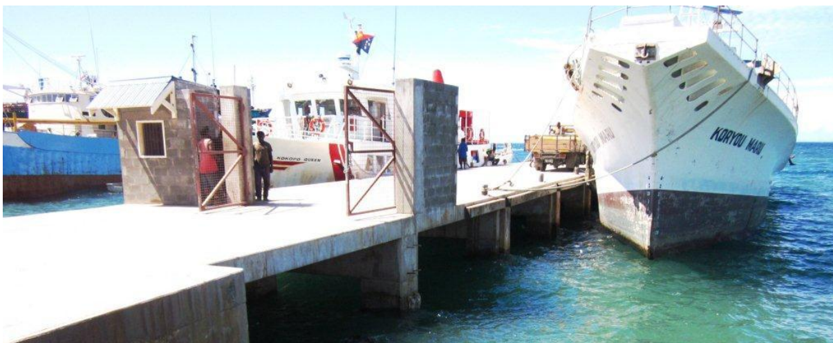
Figure 13 - Recent constructed coastal jetty
