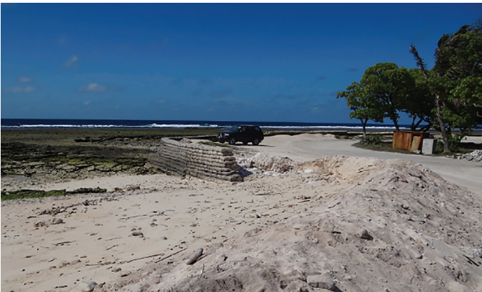
Figure 6-4 Example of a Seawall Being Outflanked in Tarawa, Kiribati
