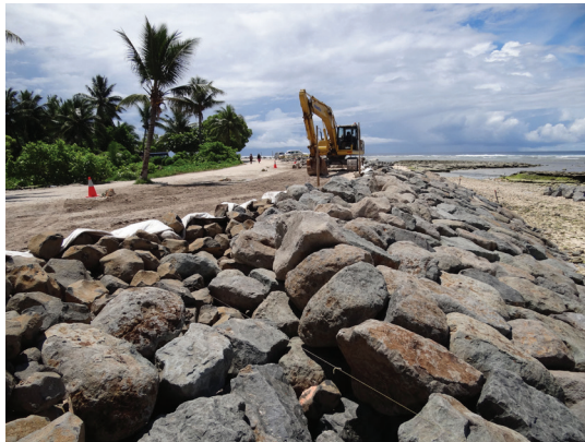
Rock revetment at South Tarawa, Kiribati
