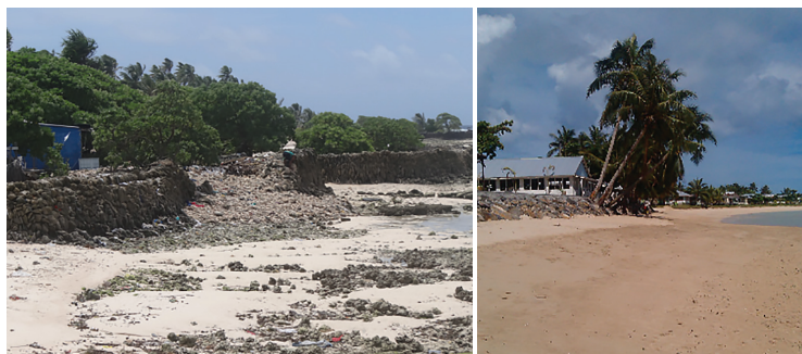
Figure 3-4 A stacked coral block wall in Kiribati collapses, forming a “Dynamically Stable Revetment” (left) and sand replenishment at Manase, Samoa (right)
