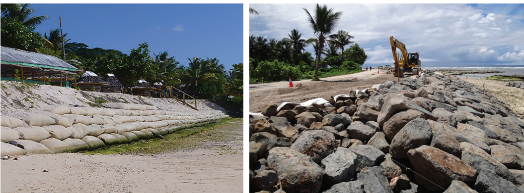
Figure 3-3 Semi-Rigid Geotextile Container at Manase, Samoa and a Rock Revetments on South Tarawa, Kiribati
