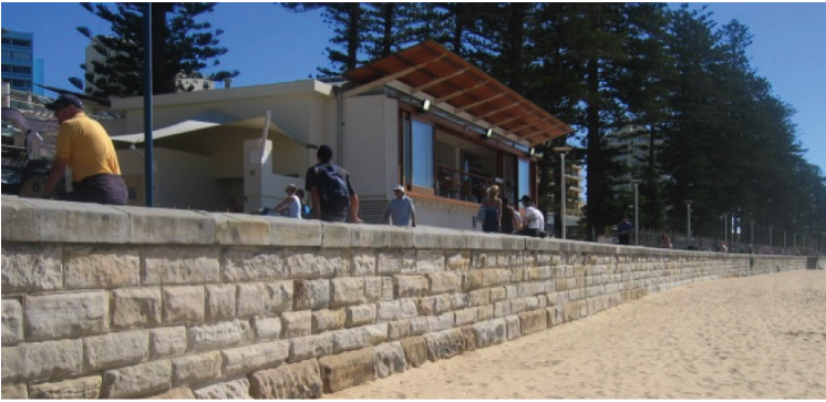
Figure 3-2 Example of a Rigid Vertical Seawall
