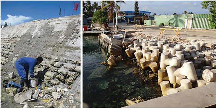
Figure 6-12 Rehabilitation of a Seawall in South Tarawa
