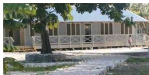
New classrooms in Kiribati. New kitset classrooms raised on timber stumps – Teeraka PS, Butaritari (2012) - the prefabricated buildings are erected by local teams
