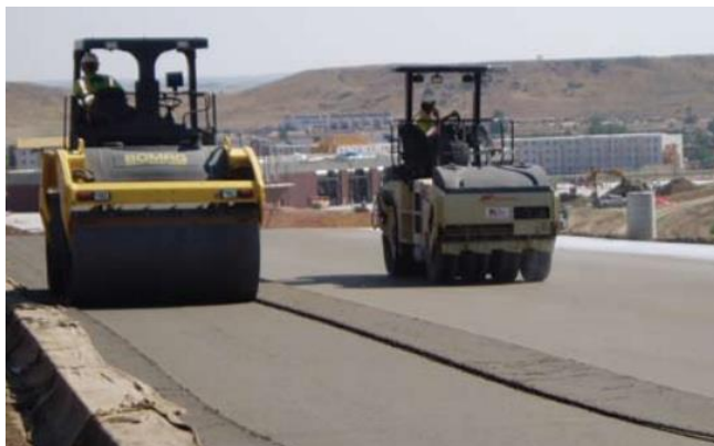
Comparison of steel drum and rubber-tired roller. (Harrington et al. 2010; p. 73).
