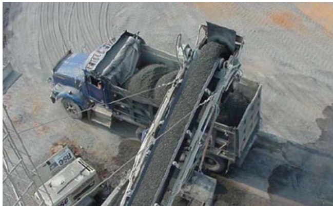
Transferring RCC from mixing plant to truck. (Harrington et al. 2010; p. 69).
