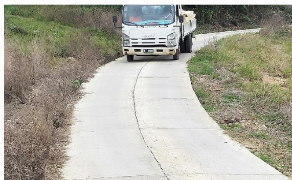
Recently constructed JCP low-volume road. Espiritu Santo, Vanuatu. (Johnson 2018b).
