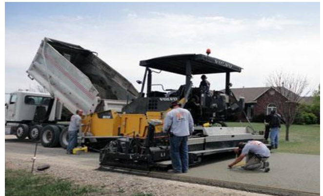
RCC loaded into paver. (Roller compacted concrete n.d).
