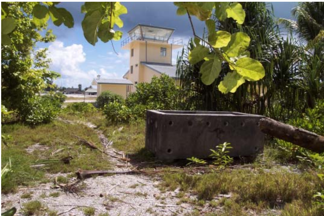
Figure 8. The septic tank toilet for the Control Tower is located over one of the infiltration gallery arms leading to Bonriki pump station 7 in the foreground right
