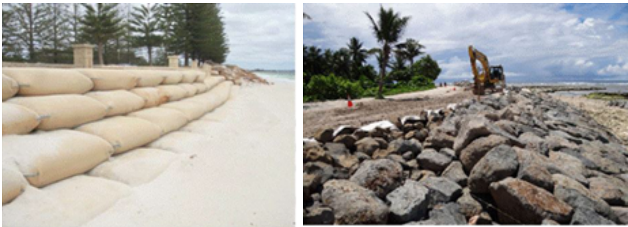
Figure 10-2: Semi Rigid Structures—Sand Filled Bags and Rock Revetments
