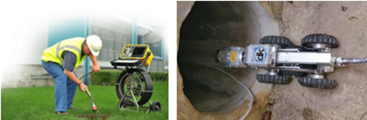
Figure 11-11: CCTV Camera Inspections of Sewer Pipes
