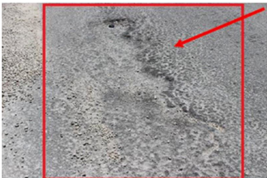
Figure 6-2: Degradation Modes of Roads—Surface Degradation Due to Ponding
