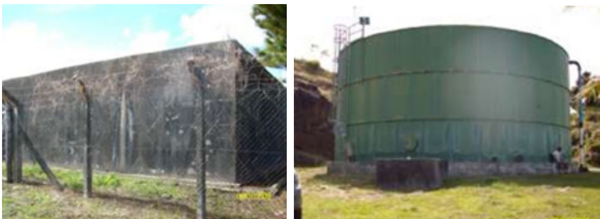
Figure 11-4: Above-Grade Water Storage Tanks (Concrete on Left, Steel on Right)
