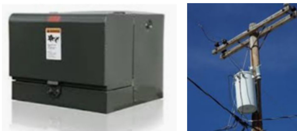
Figure 12-6: Underground and Overhead Distribution Transformers
