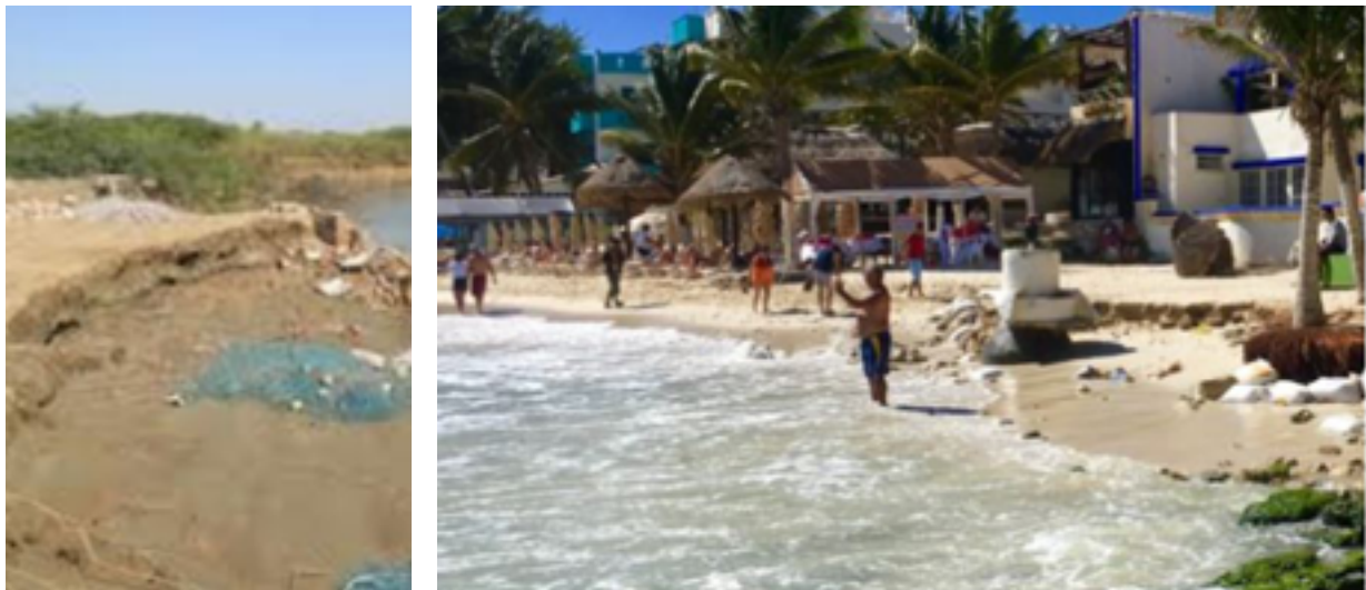
Figure 10-5: Sand Beach in “Poor” Condition due to Erosion
