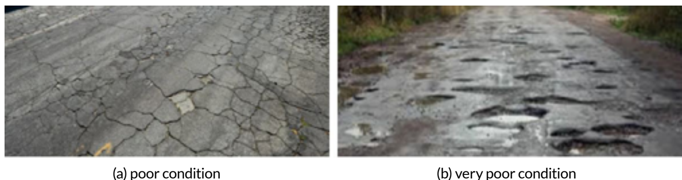
Figure 6-9: Pavement Deflection Assessments Under Load
