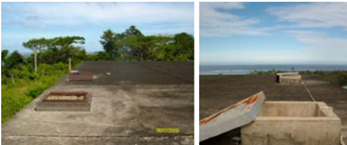
Figure 11-3: Below-Grade Water Storage Tanks with Exposed Lids
