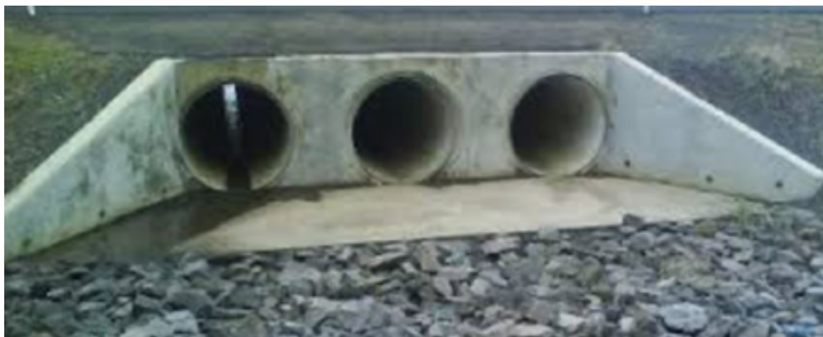
Figure 7-4: Typical Culvert
