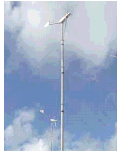
Figure 17. Two 20-kW turbines on Mangaia. (Source: Cloin and Mario, 2004)
