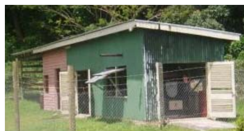
Figure 4. Generator powerhouse, Welagi Village, (Taveuni), Fiji.
