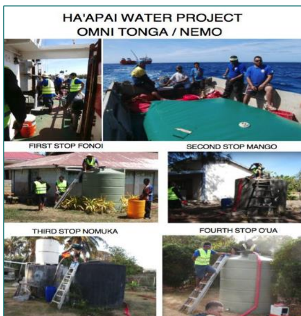
Plate 21: Ha'apai Water Project, 2014-2015
