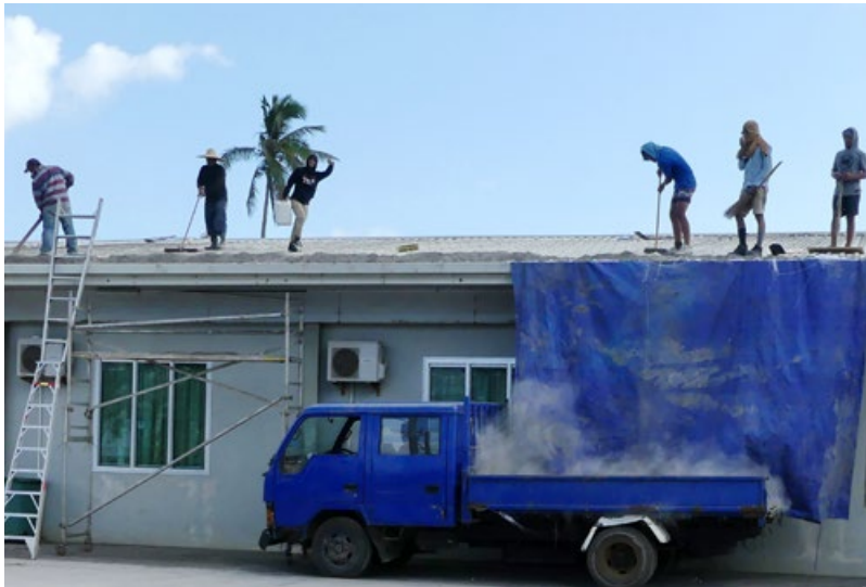
Cleaning the roof of the Ministry of Fisheries.
