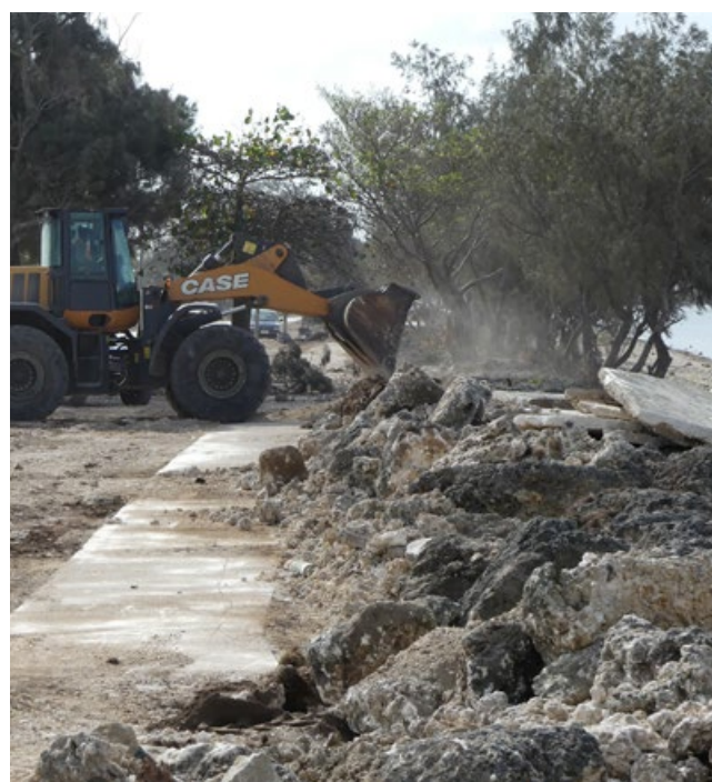
Sopu temporary rebuilding damaged seawall along Vuna road.
